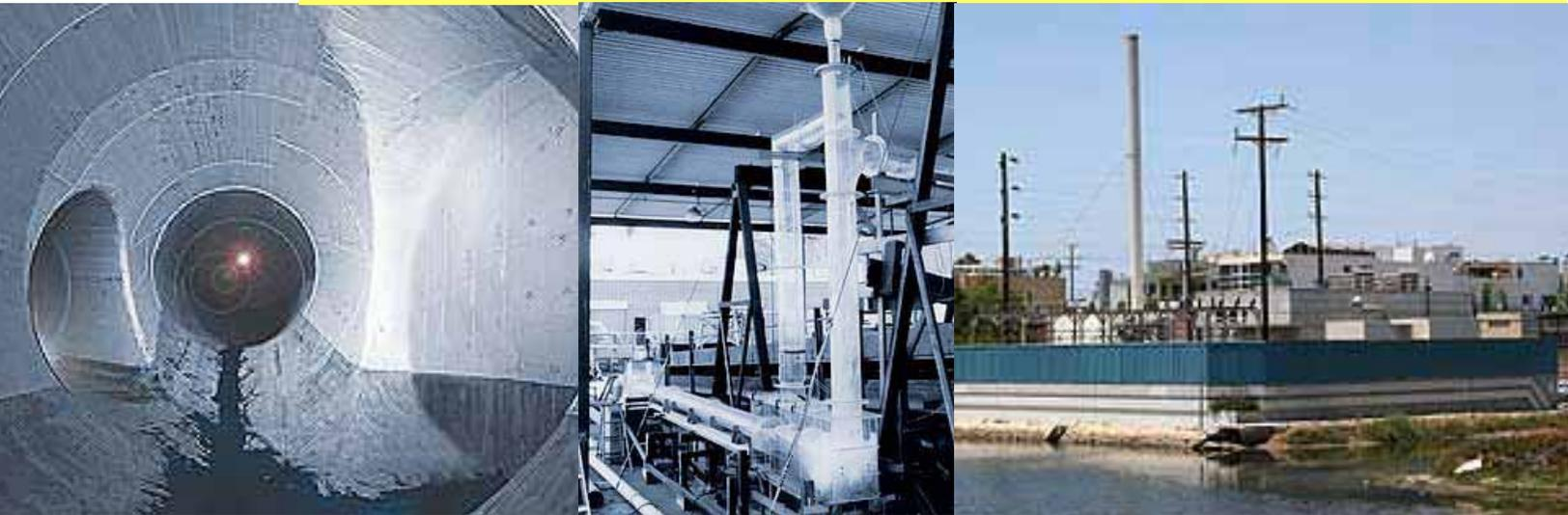
Major Components of the City of LA's Collection System: Major interceptor sewer (above left) Hydraulic model of drop structure (above center) Pumping plant (above right). Map of the City of LA's Collection System (below)
