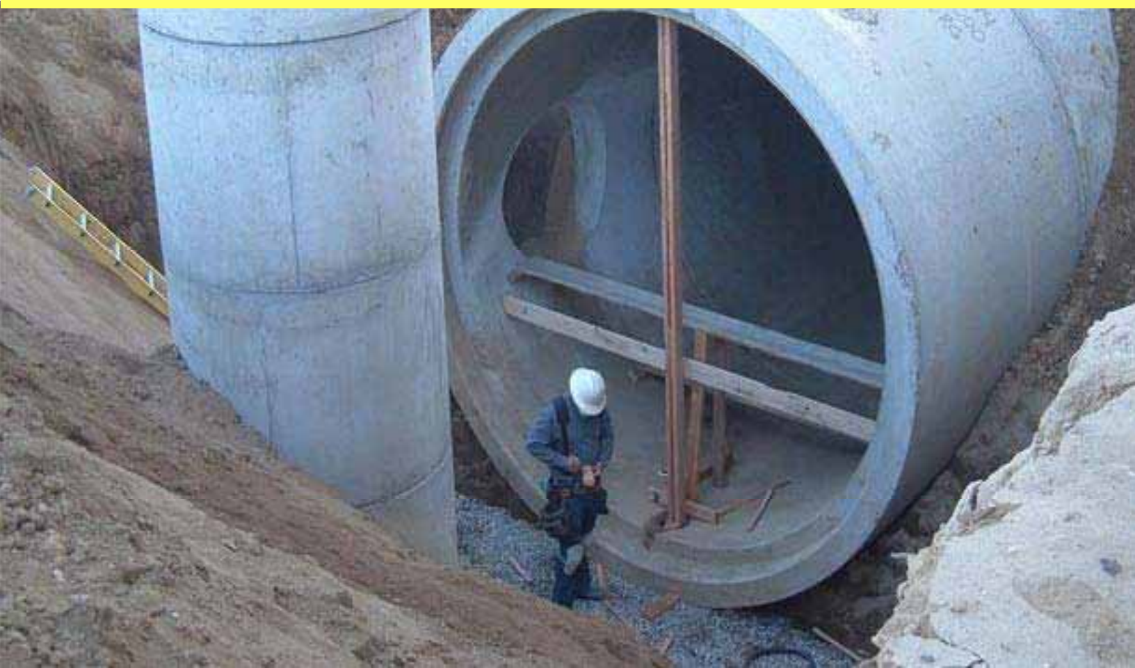
Indoor Composting Facility (above) Biofilter Header End Bulkhead Preparation (below)
