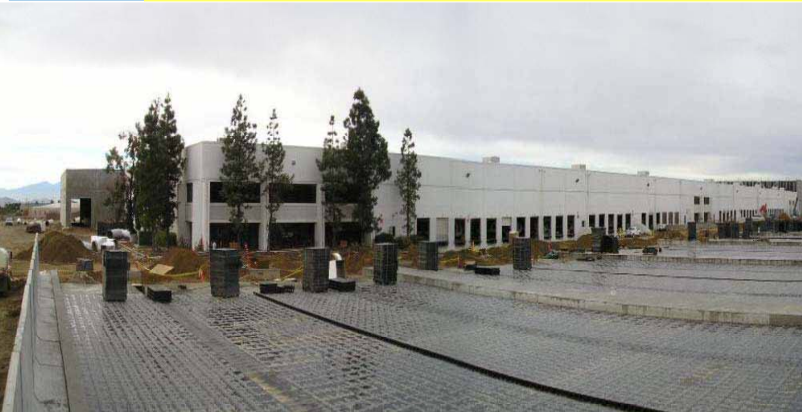
Indoor Composting Facility (above) Biofilter Header End Bulkhead Preparation (below)
