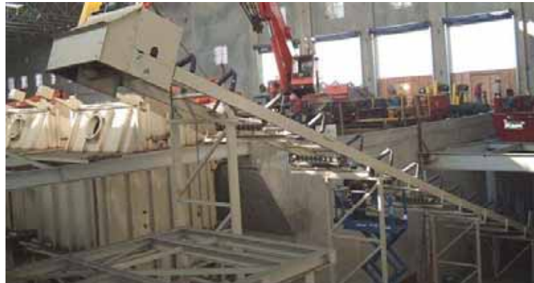
Installing conveyor support framing adjacent to biosolids hoppers
