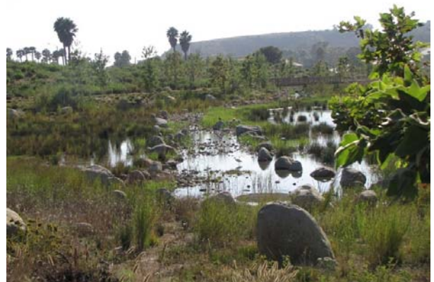
2.6 Million Gallon Detention Pond
