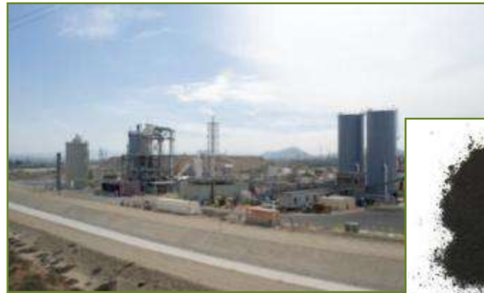
The Rialto Facility
